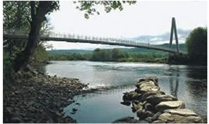
Composite footbridge built in Scotland in 1990 (top) and large carbon fiber beams from Strongwell (bottom)
