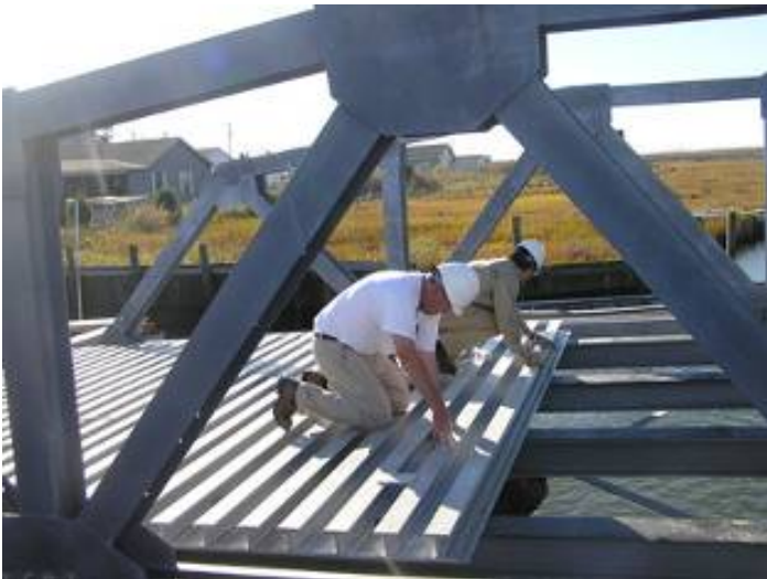
Installation of ZellComp composite bridge decking in Bradford VT (top) and Tangier, VA (bottom)
