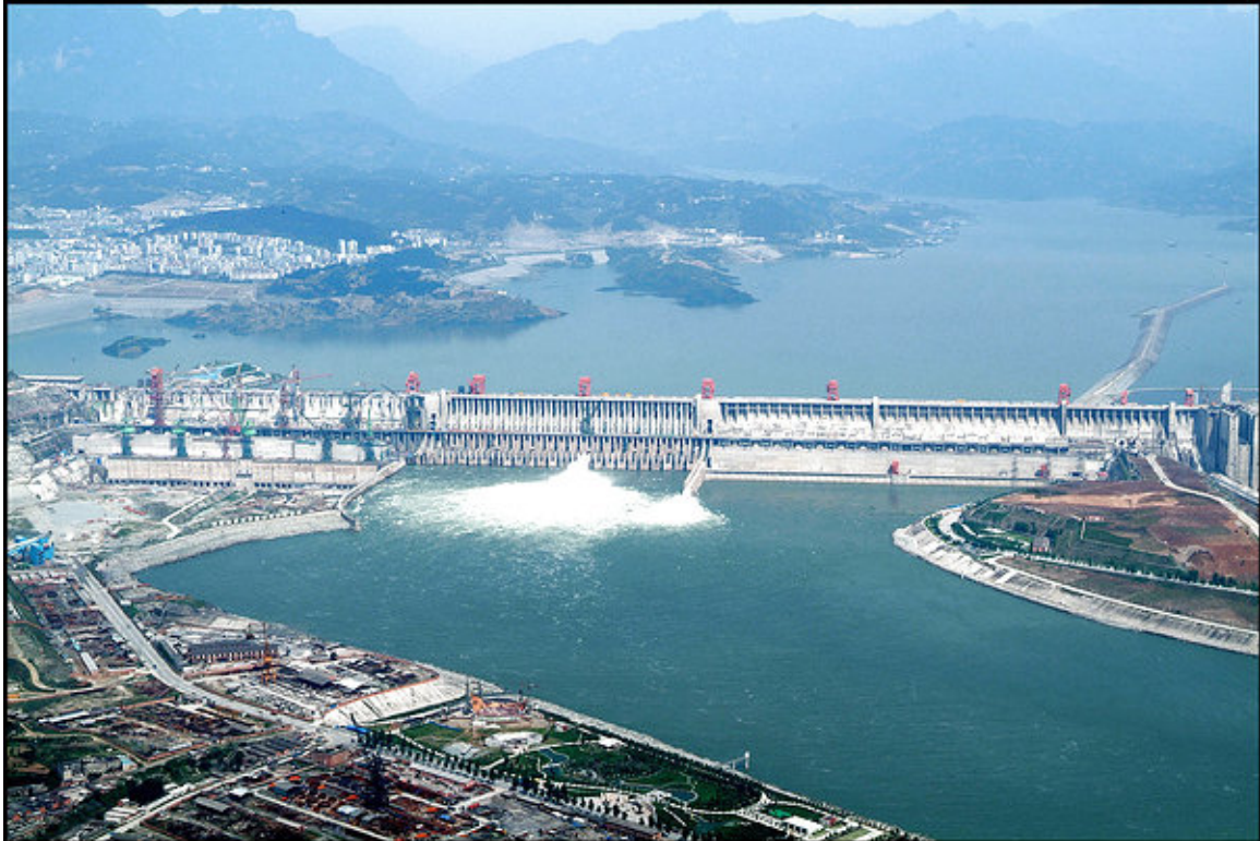
Figure 1. Large Infrastructure Projects, Such as the Three Gorges Dam in Du Huaju, China May Provide New Opportunities for Composites [New China News Agency]
